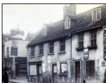
The Prince of Wales (building on left of photograph) 95
