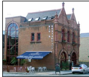
The Old Fire Station
