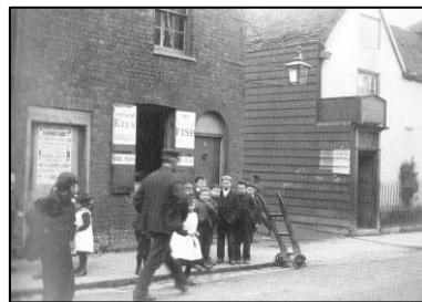
The Standard Inn before its demolition in 1897. It is the white building to the right of the fishmongers.
